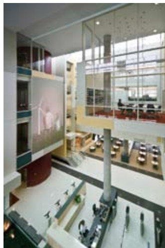
Light-filled main entry atrium and the elevated Willow Conference Room is supported by a single cast-in-place concrete column. Great River Energy produces some of the highest quality flyash pozzolana in the country
