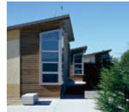
The exterior of the classroom building, featuring large north-facing windows that wrap the corner of the building to balance the light
