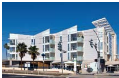
This south elevation shows the protected street-front balconies connected to day-lit living rooms. It also shows the direct access from the light rail platform to the building's street-level retail shops
