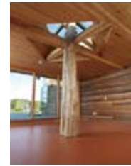
The tree-trunk column in this photograph is a feature of the classroom entry lobby. It was found at the lot of a local tree surgeon
