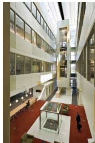
This photo highlights the building's daylight atriums, one of the strategies for providing 75 percent of the building with a minimum 25 Fc of sunlight. Artificial lighting energy is reduced by over 60 percent
