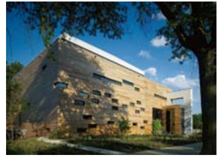
The northwest corner of the building
